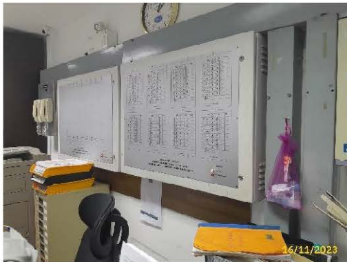
Fire Alarm Control Panel
