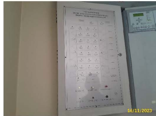
Fire Alarm Control Panel
